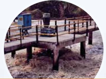
Biological Treatment Towers
