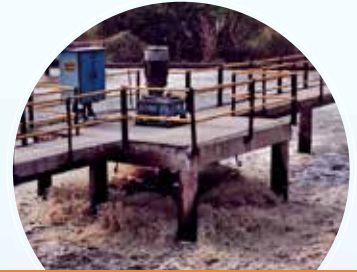
Biological Treatment Towers
